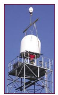
Radar network tower being installed on UMass Amherst campus
